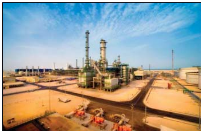
Using Sasol Ltd.'s Fischer-Tropsch process, the Oryx gas-to-liquids plant in Qatar, owned by Qatar Petroleum Co. and Sasol Ltd., will begin converting lean gas from Qatar's giant North field to products beginning in March. Photo courtesy of Sasol.
